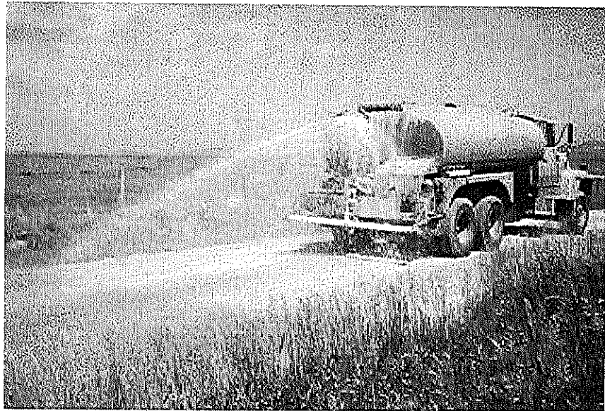
A water truck being used to prewet some very dry gravel just prior to treatment. This dramatically improves the success of the treatment.
